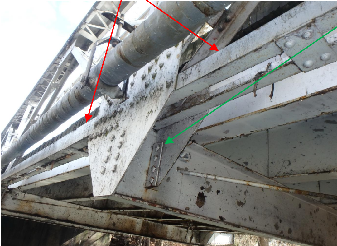
Bottom Chord Spliced at L2
