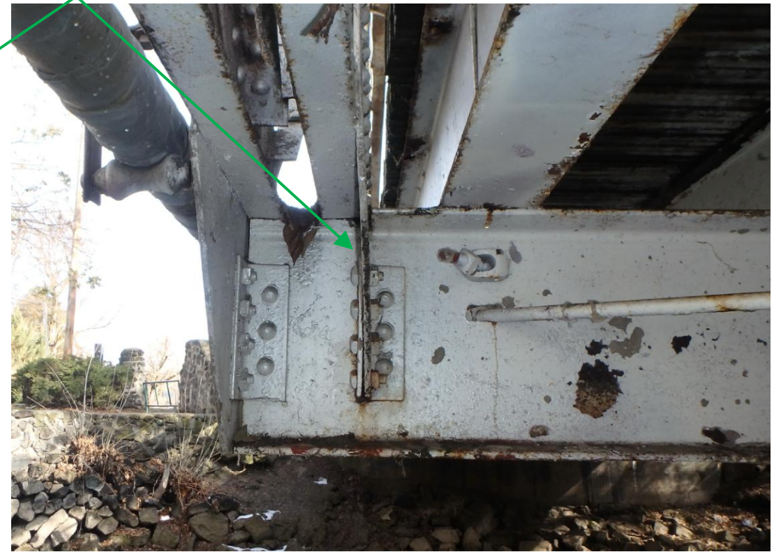
Inside Plate Slotted for Floor Beam
