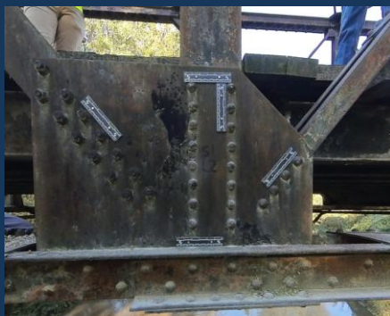
Nonstandard gusset plate details at L2 for the Iowa standard S-series trusses—S1, S2, S3, S4 and S6
