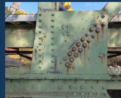
Nonstandard gusset plate details at L2 for the Iowa standard S-series trusses—S1, S2, S3, S4 and S6
