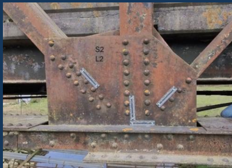
Nonstandard gusset plate details at L2 for the Iowa standard S-series trusses—S1, S2, S3, S4 and S6
