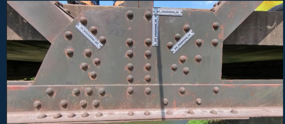
Fig. 1 Typical Iowa standard truss gusset connection
