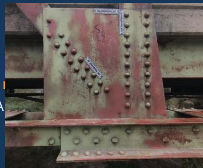
Nonstandard gusset plate details at L2 for the Iowa standard S-series trusses—S1, S2, S3, S4 and S6
