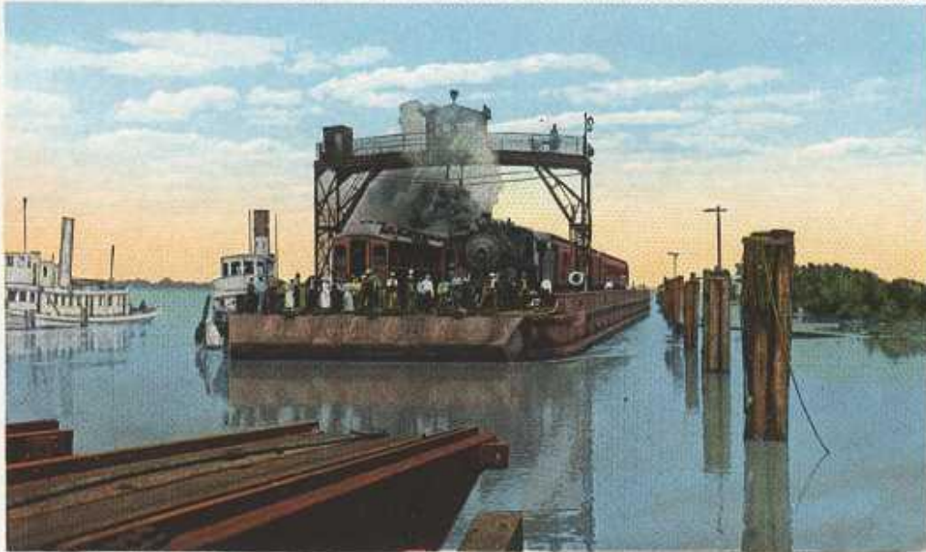
CROSSING MISSISSIPPI RIVER AT AVONDALE, TEN MILES ABOVE NEW ORLEANS, LA.
