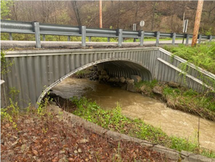
Figure 3. Metal Culvert
