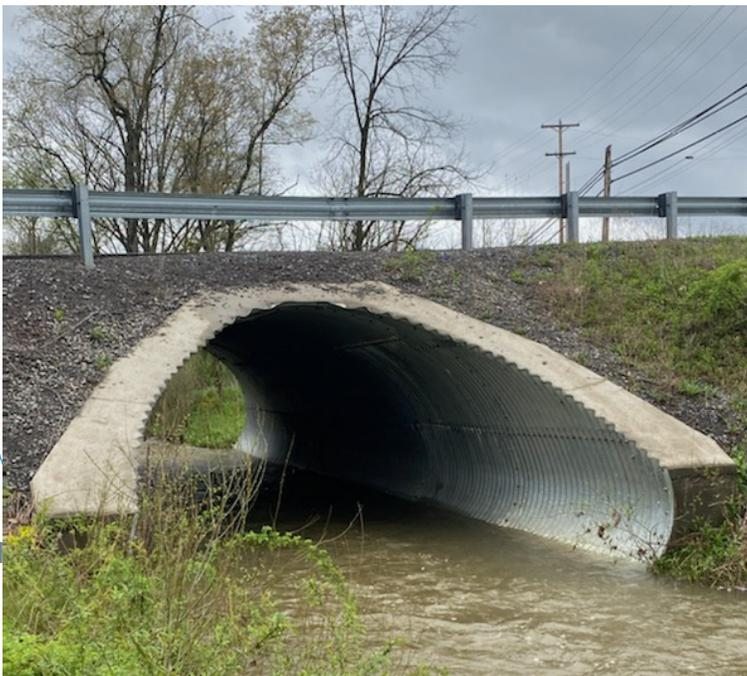
Figure 4. Metal Culvert
