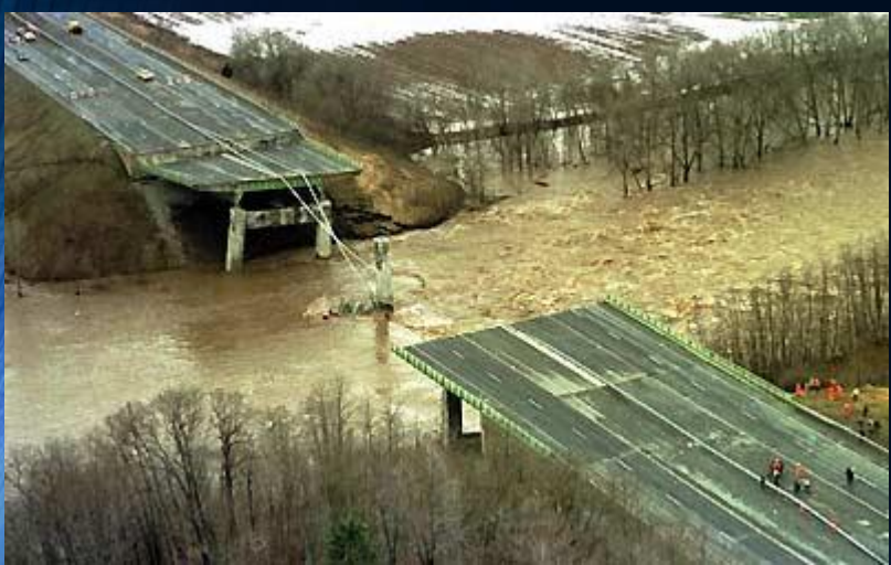
Built 1954, Collapsed April 1987
