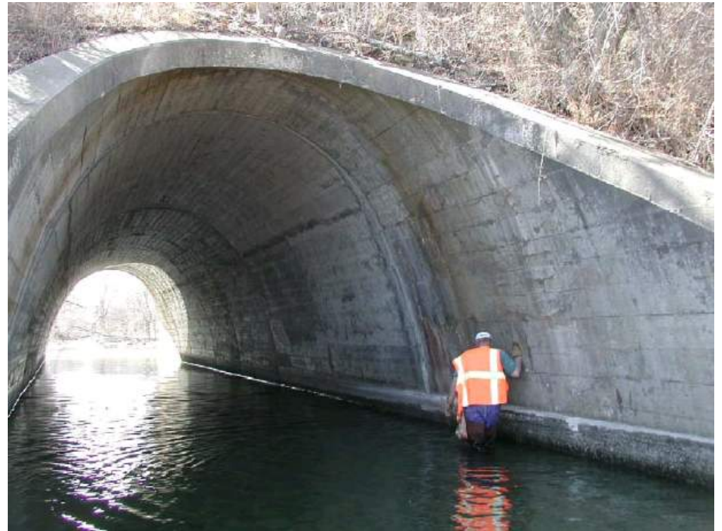
Reinforced Concrete Filled-Spandrel Arch
