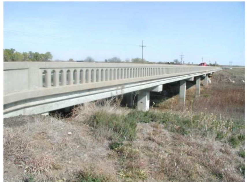
Continuous IBS Bridge
