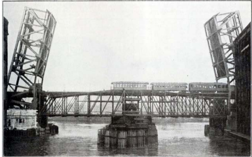
OLD AND NEW DRAWBRIDGES OVER THE CHICAGO RIVER AT LAKE ST.
