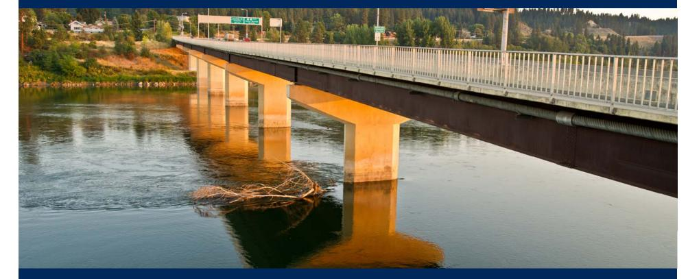
Load Rating of the Bonners Ferry Bridge: A Case Study of Evaluating Post-Tensioned SteelGirders
